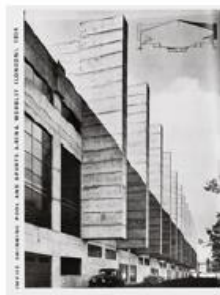
4. Empire Pool, view of concrete counterweighted trusses
