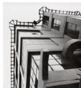
5. Sainsbury Warehouse, London, 1931–33, cross section and view from below showing the track for the window-cleaning cradle -pp. 138–139-
